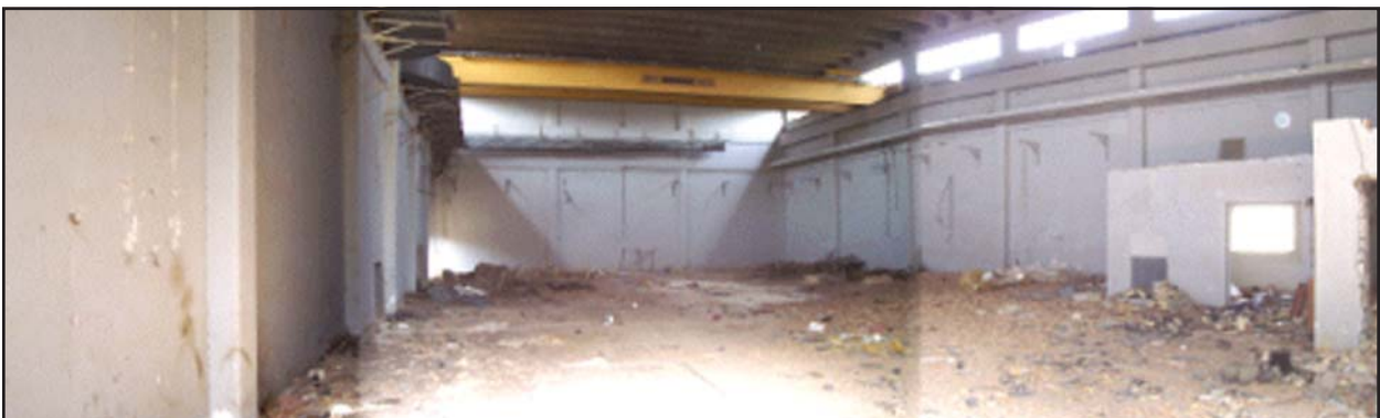
Figure 8. Al Hamath facility.
