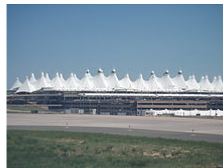
The Teflon-coated fiberglass roof of Denver International Airport resembles the Rocky Mountains .
